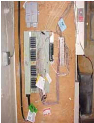
Existing Telephone Wiring Termination Installation
