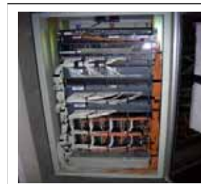
New network installation at an Adult Education and Occupational Center
