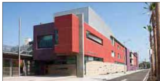
East Valley Area New MS #1 - Completed
