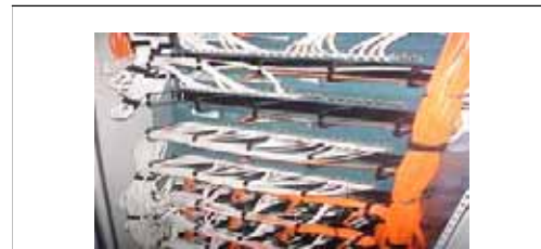
New LAN Installation
