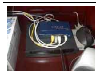
Old EEC Network Installation
