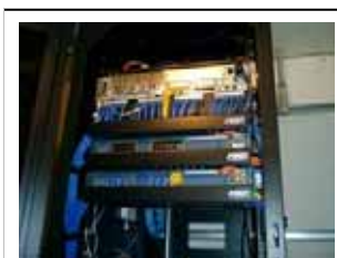
New EEC Network Installation
